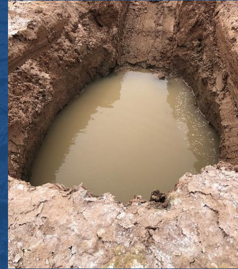
Trenching and brine close to surface
